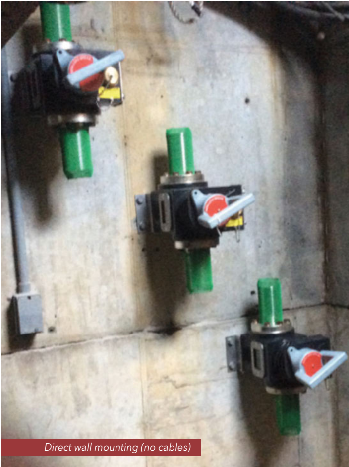
Load-side bottom installation shown with submersible non-energized cap
