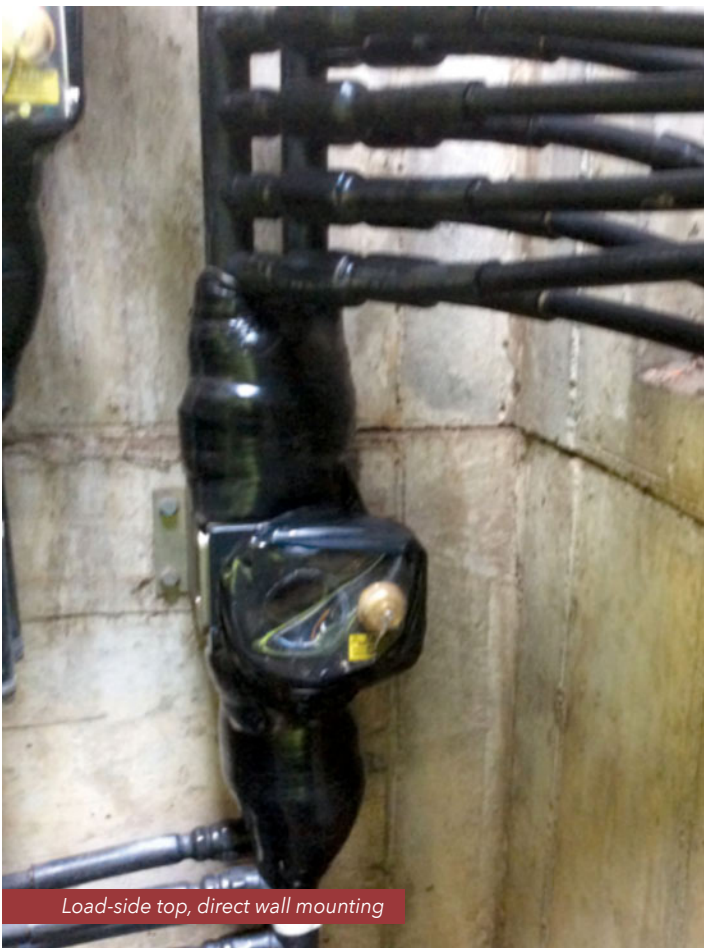
Direct wall mounting (no cables)
