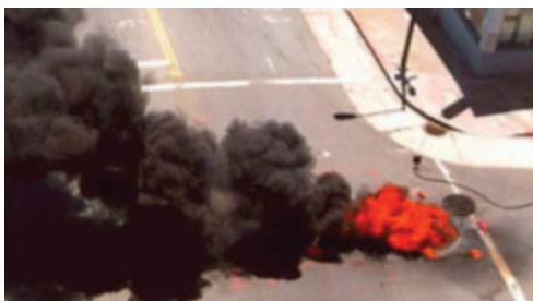
Transformer Vault Explosion & Fire
