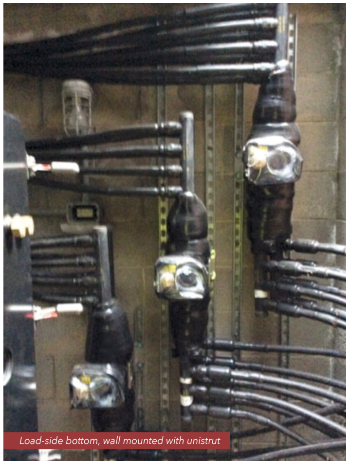
Load-side bottom installation shown with submersible non-energized cap
