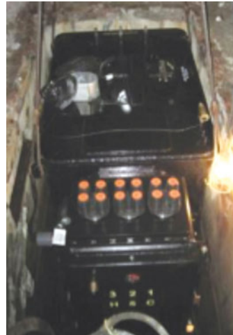
Low Profile Submersible Dry-Type Transformer
