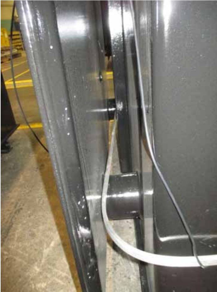
Ribbon anodes for radiator panels
