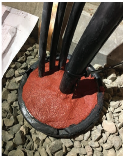
Effective seal 1 One part sealant
