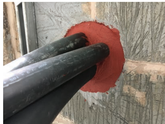
Effective seal 2 One part sealant
