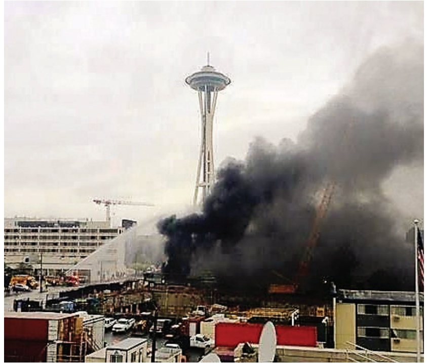
Broad Street Substation Fire
