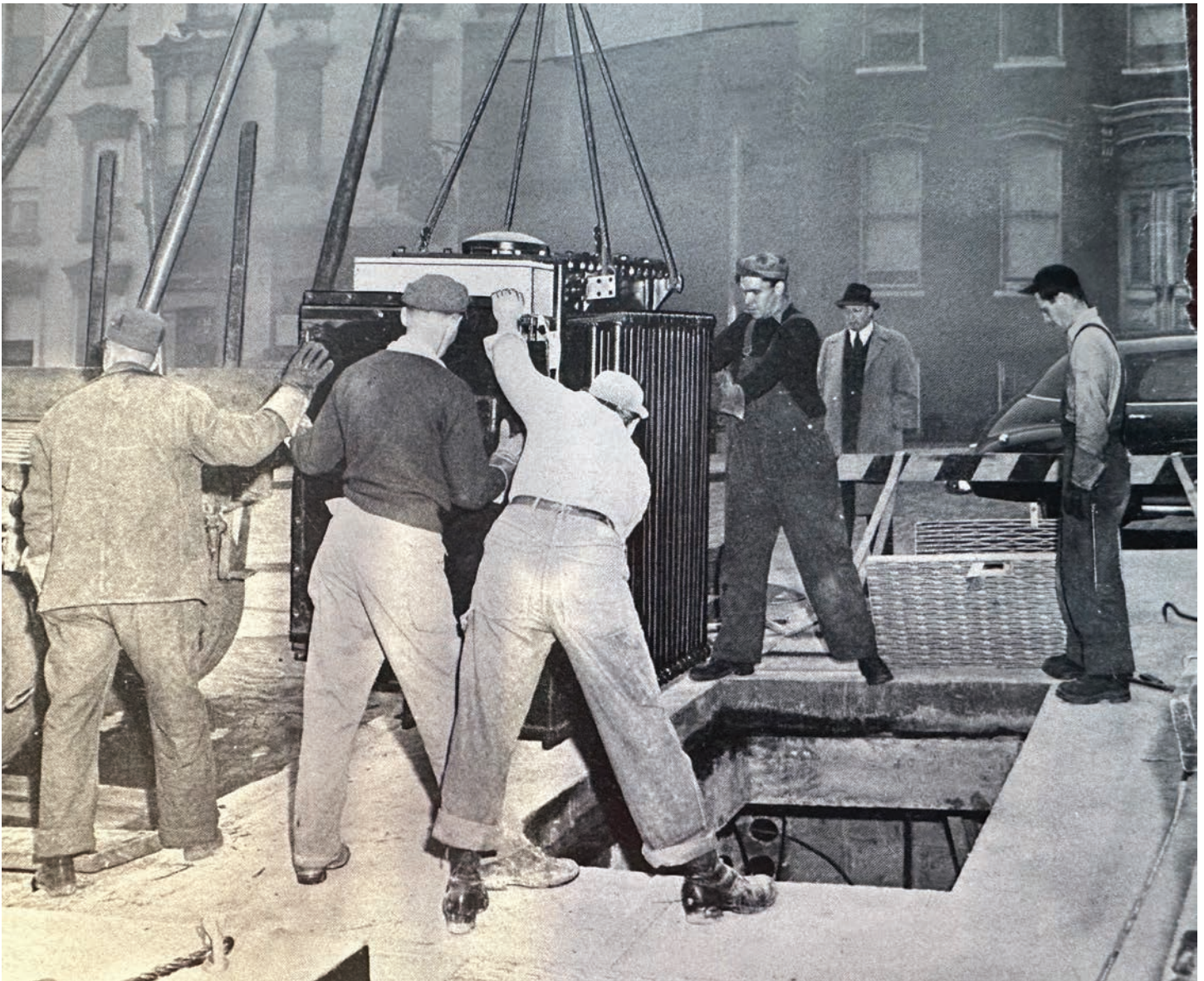
Photo 4: The lowering of an early Network Transformer
